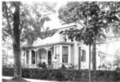
Above: The McCracken family home at 409 West Madison Street, ca. 1900.
